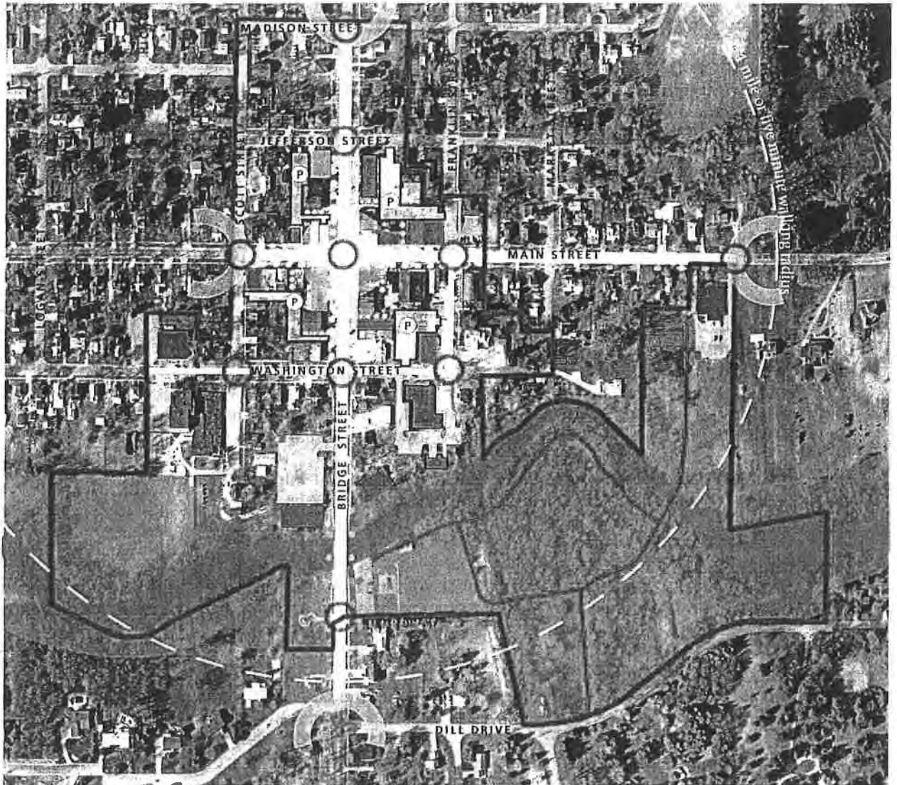
Aerial photograph manipulated by PBI to reflect new construction
